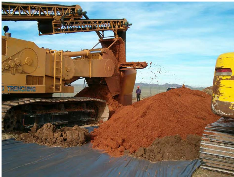
Figure 5.2 Laying Excavated Trench Soil on Plastic Sheetting, Altus AFB, Oklahoma
