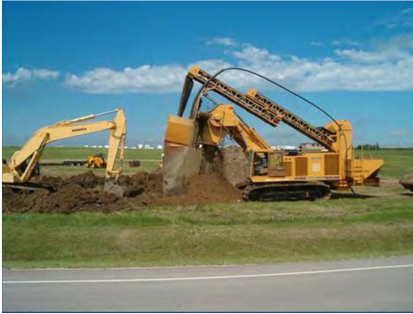
Figure 3.6 Continuous Chain Trencher at Ellsworth AFB, South Dakota
