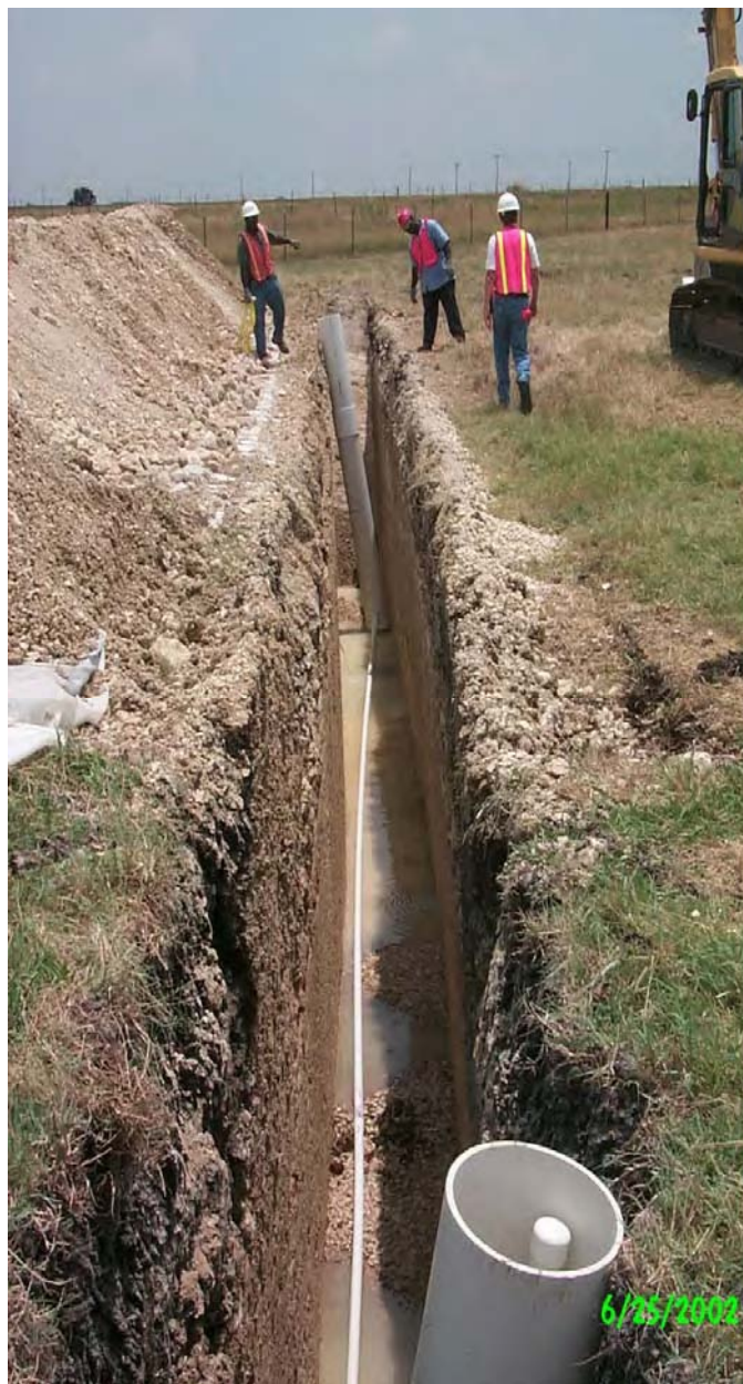
Figure 3.7 Installation of Vertical Injection Risers and Horizontal Pipe at NWIRP McGregor, Texas (photo courtesy of US Navy)
