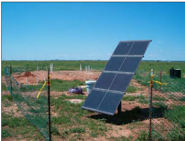
Figure 2.1 Solar Panel to Power an Extraction Pump for the Remote Bioreactor Site at LF-03, Altus AFB, Oklahoma
