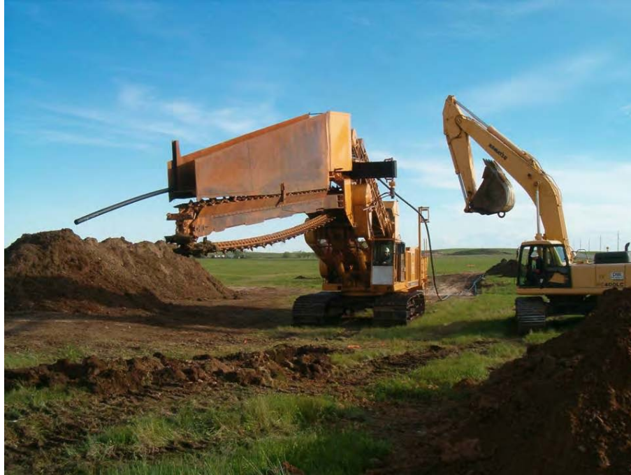
Figure 4.2 Slotted HDPE Pipe Threaded Through a Continuous One-Pass Trencher Prior to Installation, Ellsworth AFB, South Dakota
