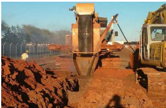
Figure 1.1 Installation of a Permeable Mulch Biowall at Altus AFB, Oklahoma
