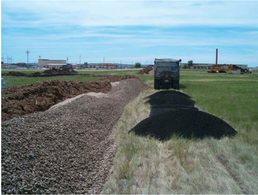
Figure 4.1 Stockpiling of Biowall Materials Prior to Mixing at the BG-05 Site, Ellsworth AFB, South Dakota (from left to right is mulch, sand, gravel, and magnetite ore)
