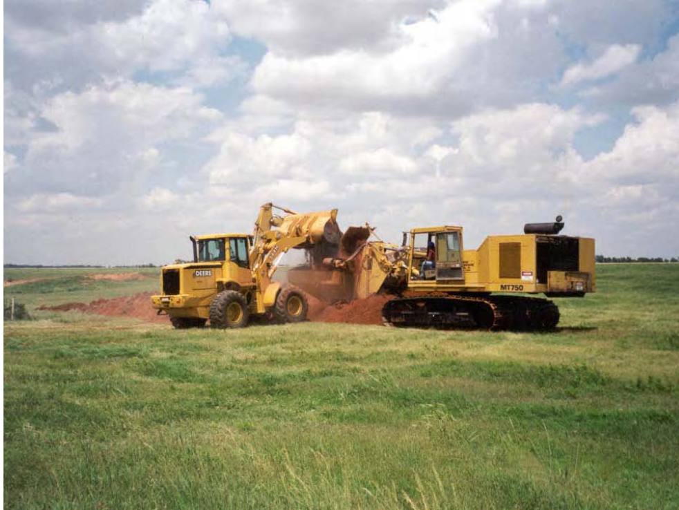
Figure 3. LF-03 Biowall Installation Using a Continuous One-pass Trencher
