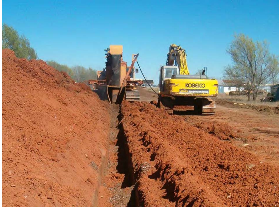
Figure 5.1 Laying Excavated Trench Soil in a Windrow Along the Biowall Alignment, Altus AFB, Oklahoma
