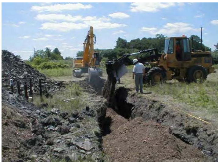
Figure 3. Installation of the Ash Landfill Biowalls
